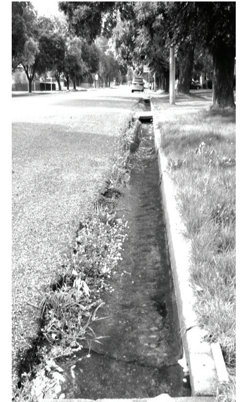
An example of formerly agricultural irrigation systems using city street gutters as their distribution network in Logan, Utah.
